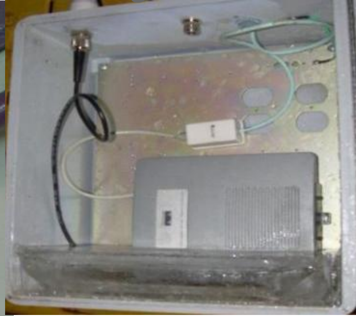
Outdoor NEMA box not weatherized (just keeping the packets on ice)
