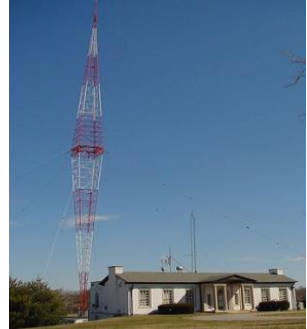
808 Ft Broadcast Monopole WSM 650 AM (erected in 1932) Nashville Tennessee - Grand Ole Opry
